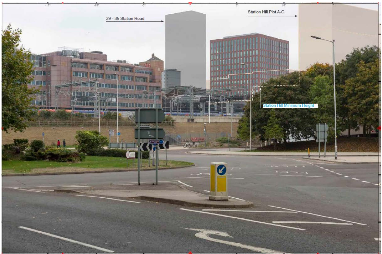
Verified view from Reading Bridge looking south-west
